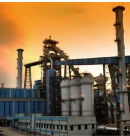
DANIELI CORUS BLAST FURNACE
